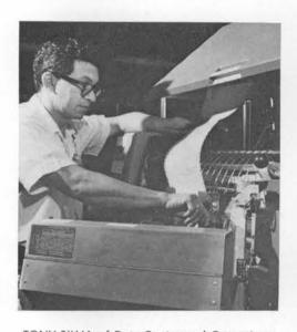
TONY SILVA of Data Center and Operations Department prepares an IBM 1401 computer printer to run paychecks. Printing operation is controlled by the output tapes from the 7090 computer.
